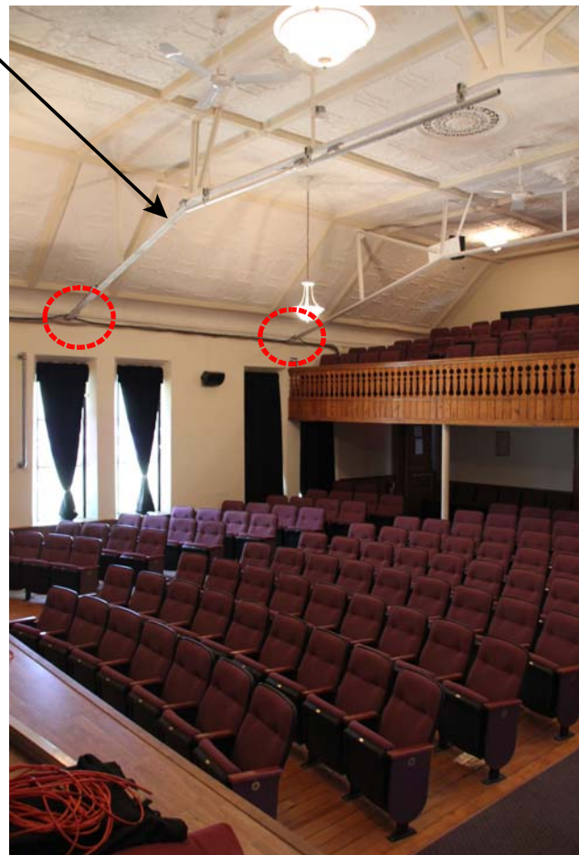
Performance Hall auditorium with exposed portion of steel trusses at ceiling.
