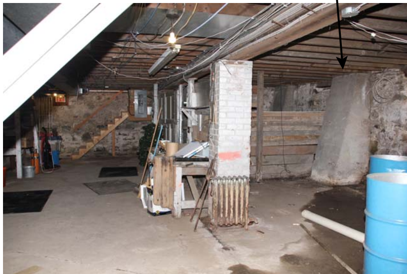
Basement, looking south.
