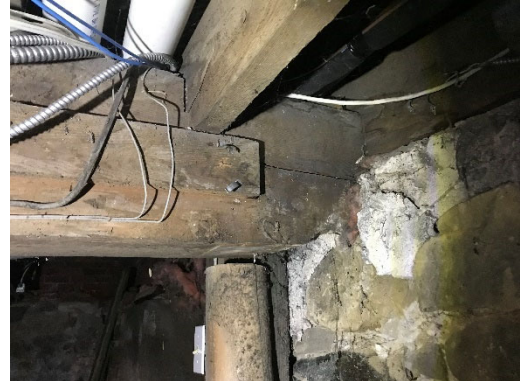
North Wall Beam Bearing
