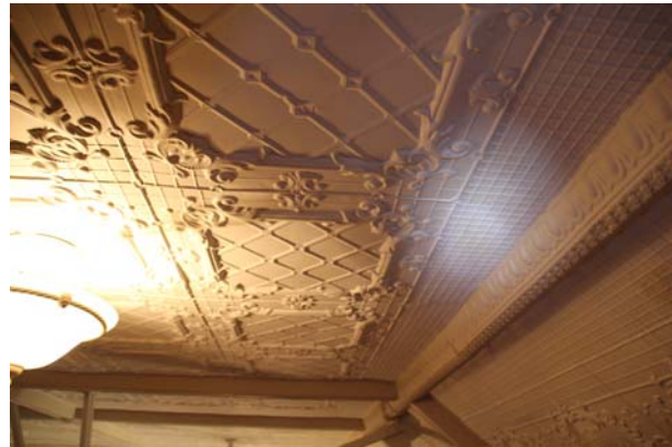
Decorative pressed metal ceiling at performance hall.
