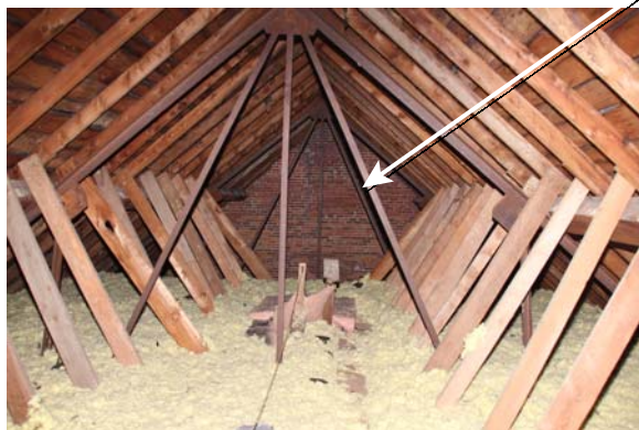
Attic above auditorium, looking north.
