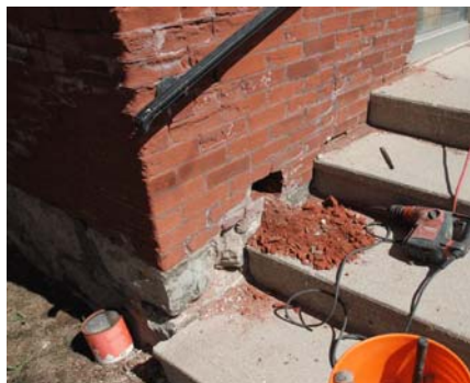
Observation port at west side of stairs.
