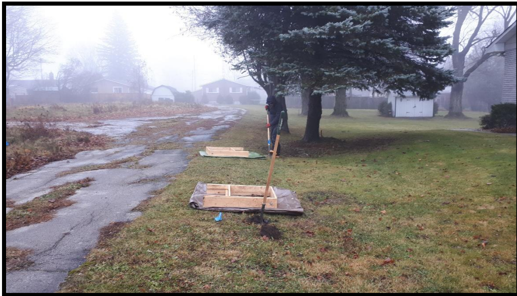
Image 4: Test Pit Survey (Facing Southeast)
