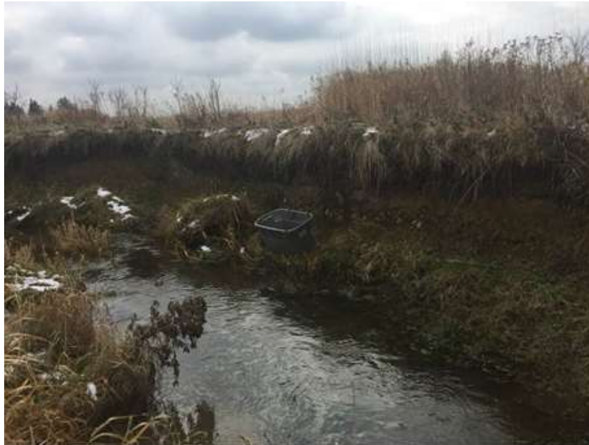
Plate 5: View of slumping shoreline of James Foley Drain downstream of the bridge at Ida Street.
